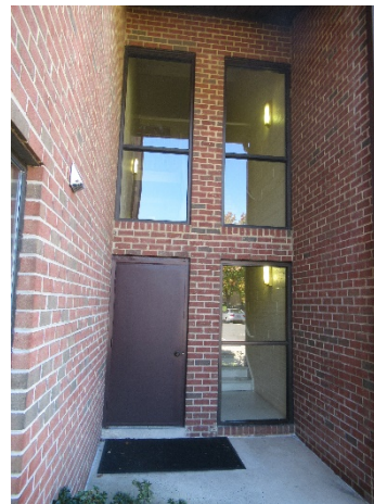
Common windows and door overview
