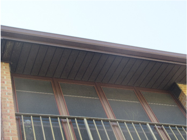
Aluminum soffit overview
