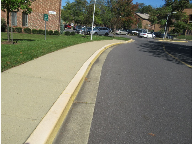
Concrete curbs and gutters overview
