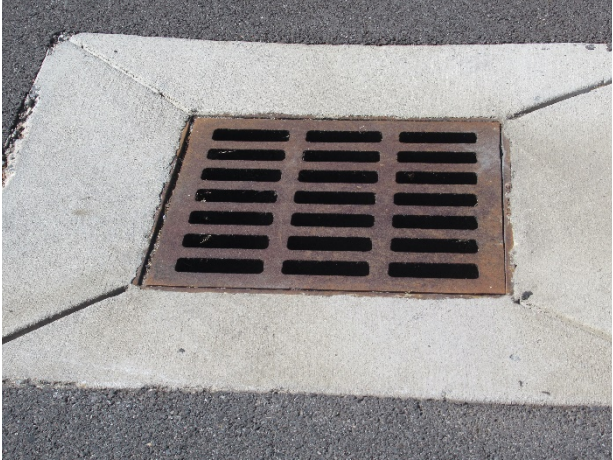
Catch basin overview
