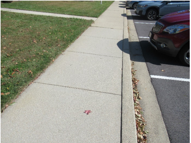
Concrete sidewalk overview
