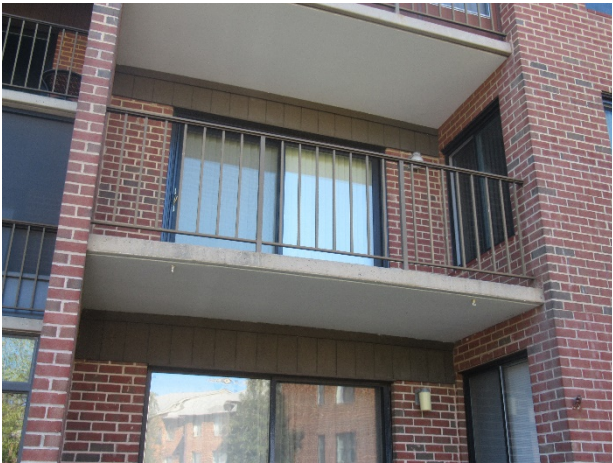
Concrete balcony overview
