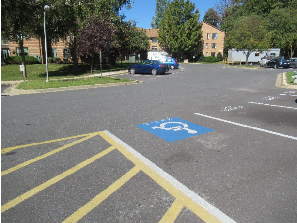
Asphalt pavement overview
