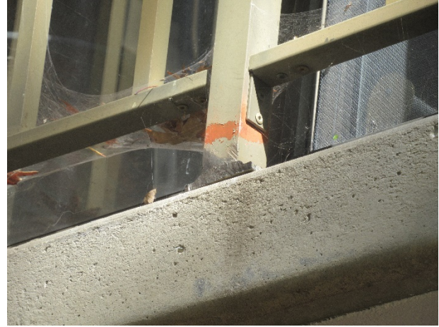
Finish deterioration
