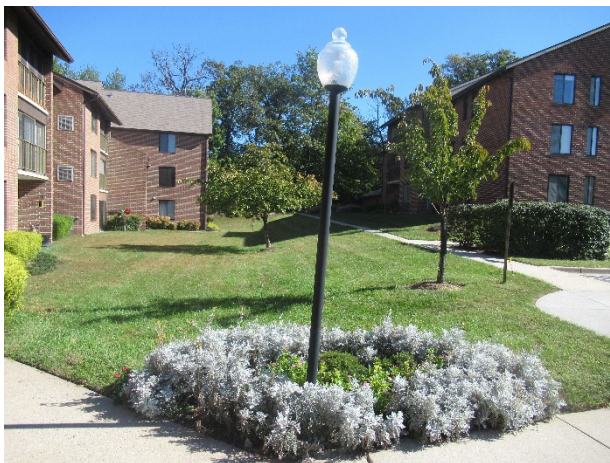
Light pole and fixture overview – Note: lean
