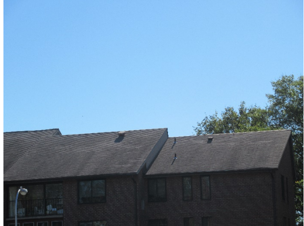
Remaining roofs overview
