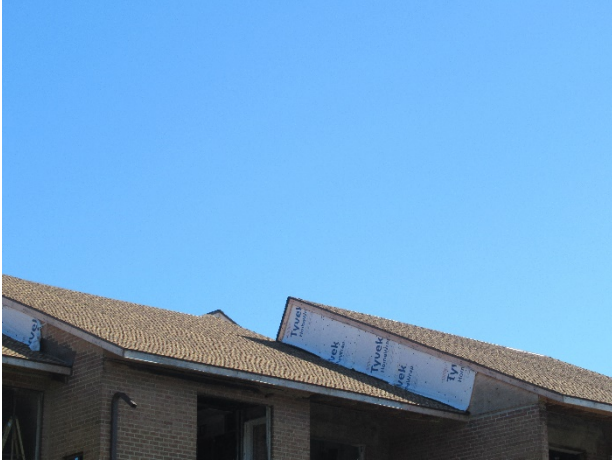
Building 91 roof overview
