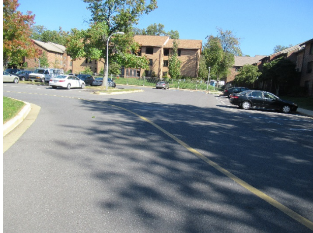
Asphalt pavement overview
