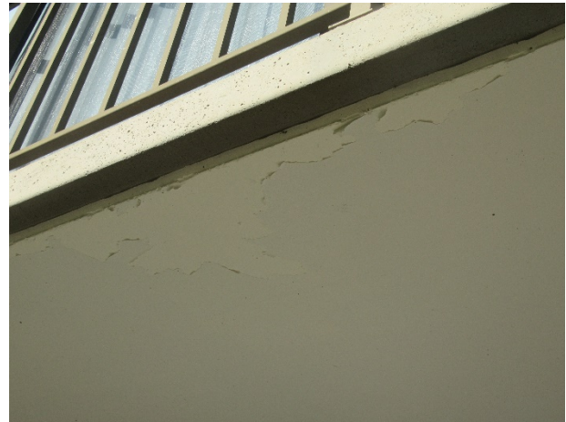
Finish deterioration
