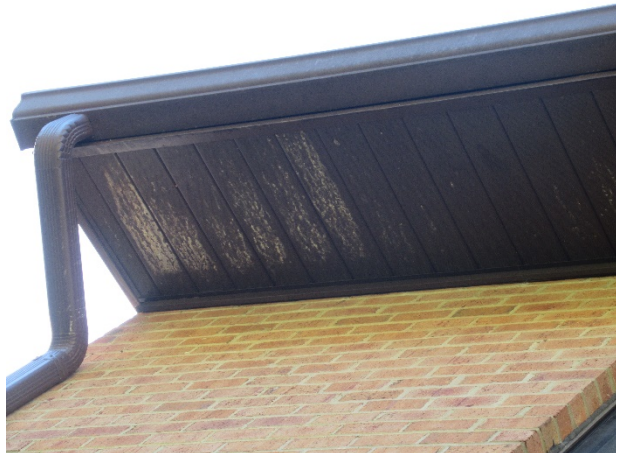
Finish deterioration
