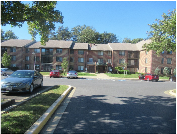
Front elevation overview
