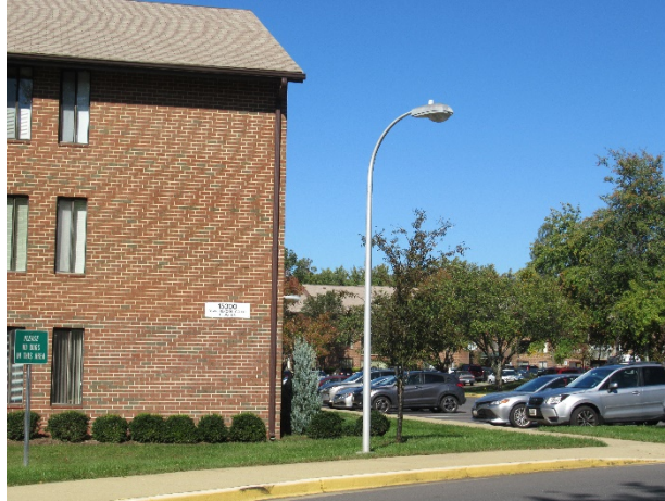
Parking areas light pole and fixture
