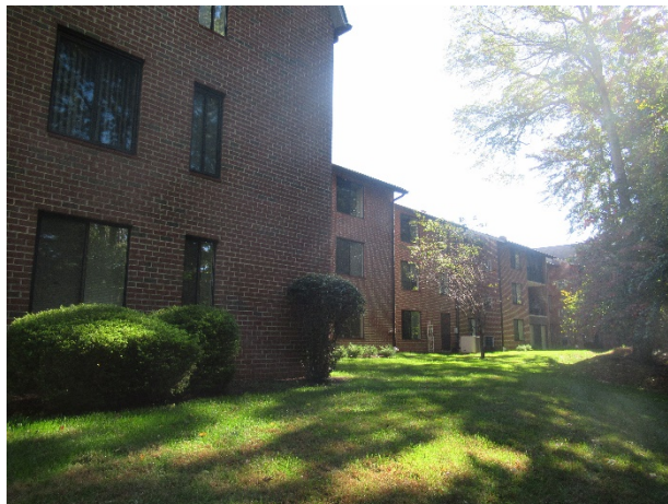
Rear elevation overview
