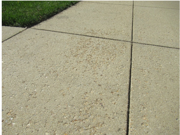
Concrete scaling
