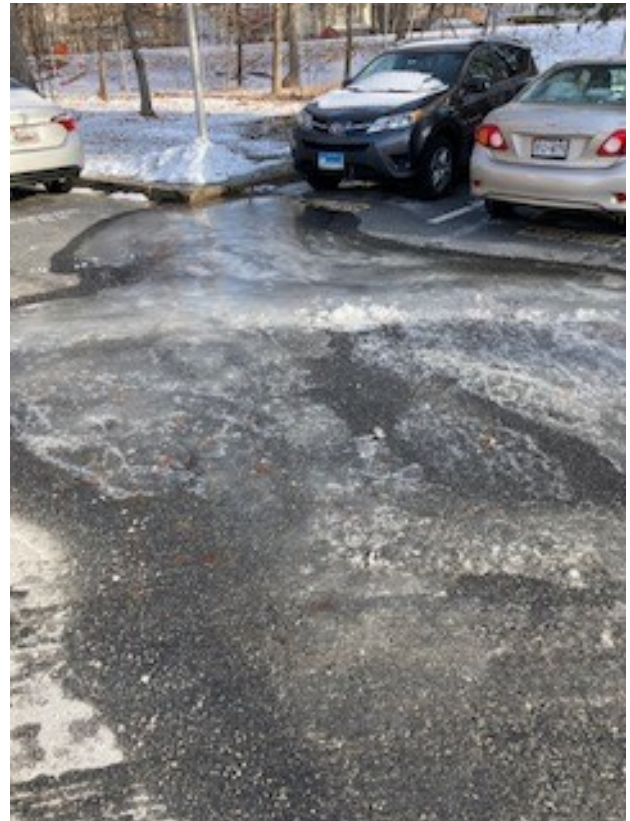
View From Bldg 93 + 94 Towards Grassy Area
